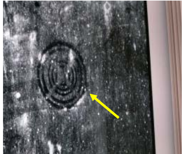
Photo Above shows an installed window with heavy condensation on Glass. Different patterns are visible within the condensation including the outline of a Vacuum Cup mark which may have been used to handle the glass during fabrication or installation. There are no visible marks present on this glass in the absence of condensation.
