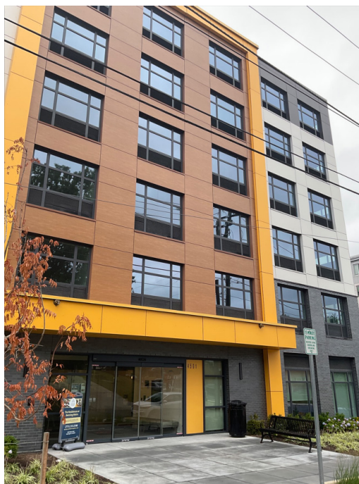
Figure 14: Photo of 4501 Blaine Street NE Taken by DOB Inspector at Certificate of Occupancy Inspection on August 19, 2025.
