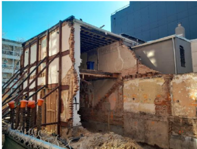
Figure 8: Rear View of 1113 V Street NW Construction Site
