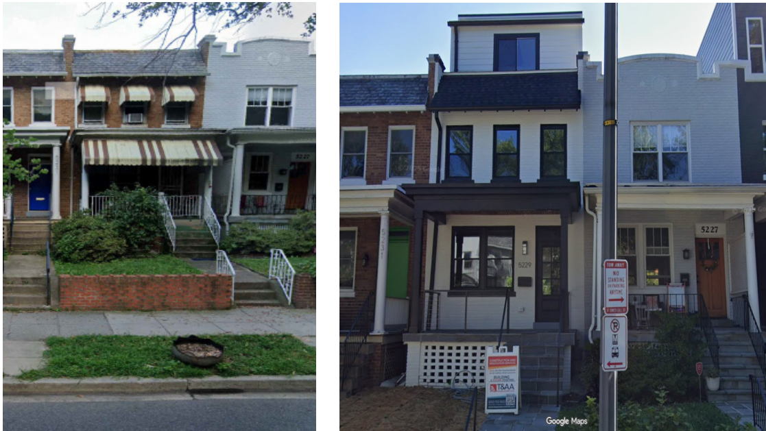
Figure 11: 5229 5 th Street NW Before Construction and After Construction
