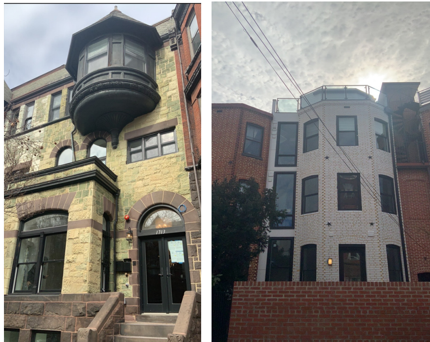
Figure 9: Photos of 1713 Q Street NW taken by DOB Inspector at Certificate of Occupancy Inspection on February 18, 2025 (left is front view; right is rear view)
