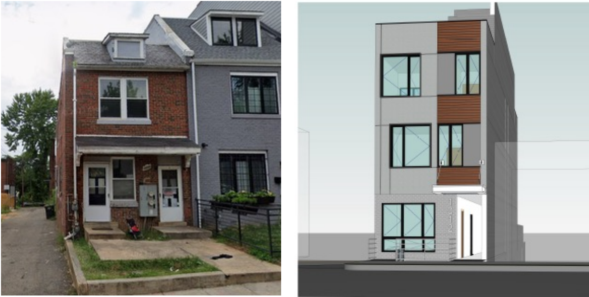
Figure 12: 1012 17 th Place NE Before Construction and Photo from Plans Submitted to DOB
